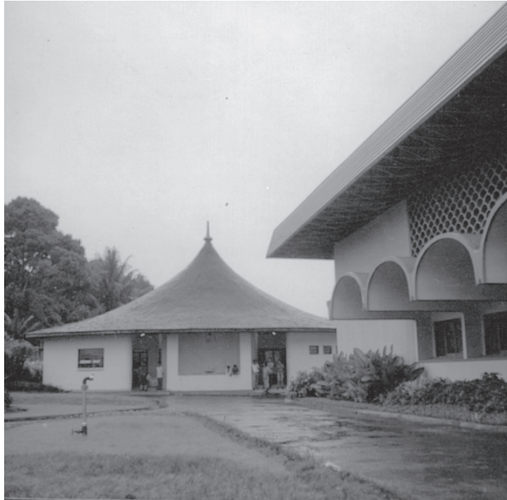
Nattermann pharmaceutical factory designed by Ramzi Winkler IDC
