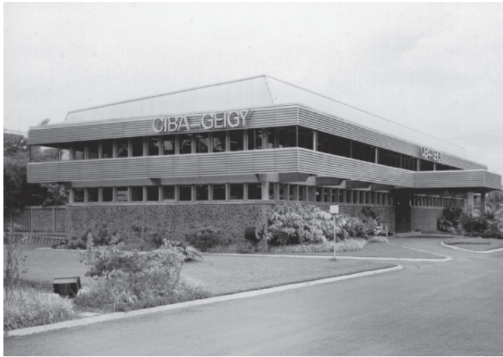
Ciba Geigy pharmaceutical factory designed by Lambert Gibbs, IDC
