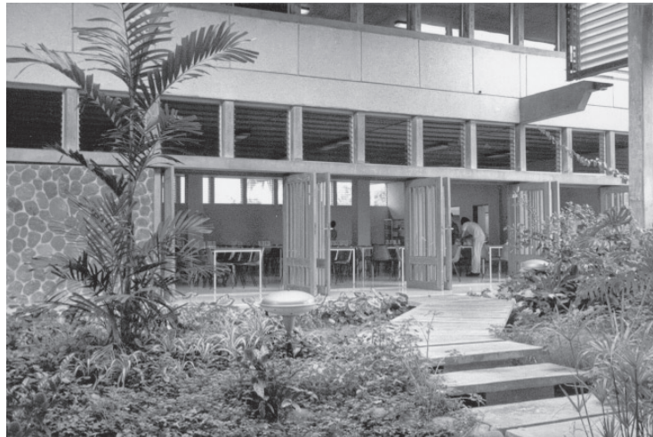
Ciba Geigy office and employees' canteen
